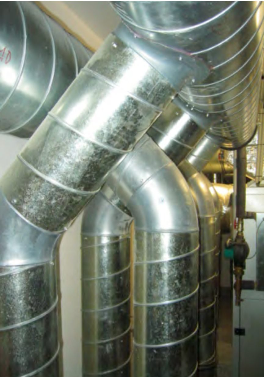
Spiral wound galvanised steel – Efficient, robust, cleanable. Photo: Alan Clarke
