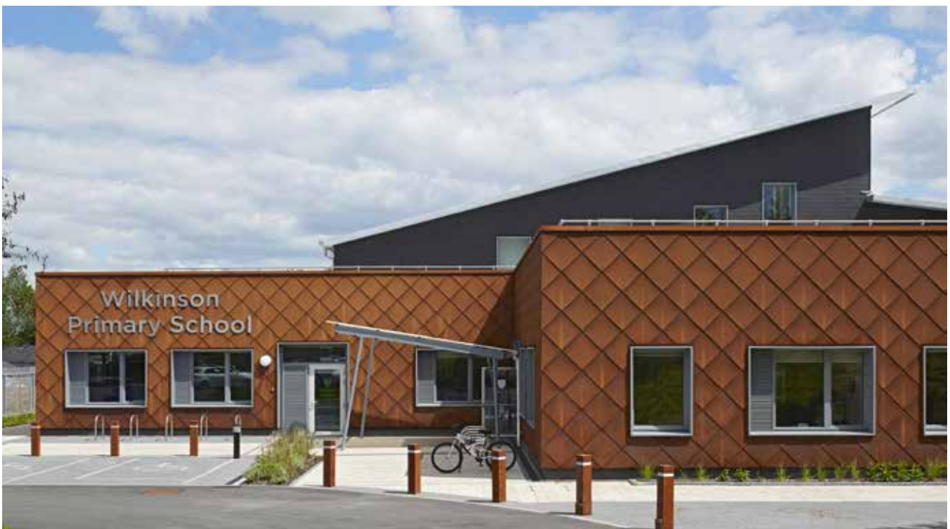
BELOW: Wilkinson Primary School, Photo: Architype
